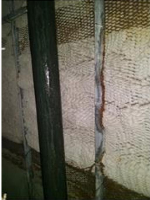
Missing insulation on cold water riser
