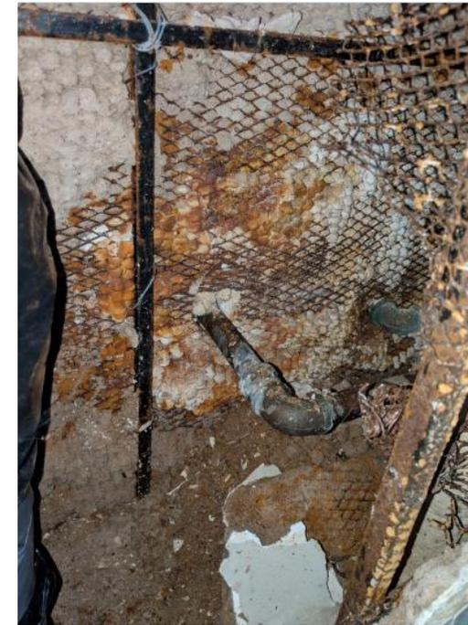
Missing insulation on cold water supply t
