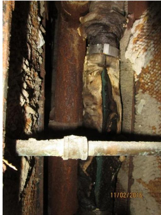
Damaged insulation on cold water riser
